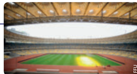
The Olympic Stadium in Kyiv
