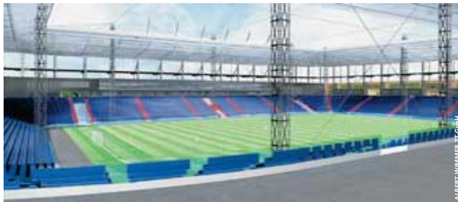
Work has started at Salzburg's stadium.
