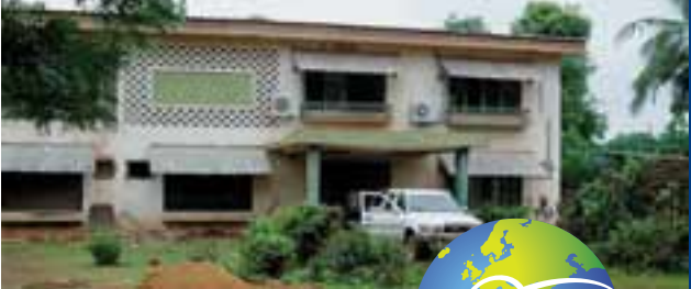
The building which will house the FA of the Central African Republic.
