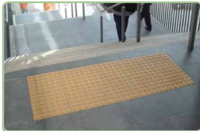
Figure 8 – A tactile wayfinding surface indicating a change in level
