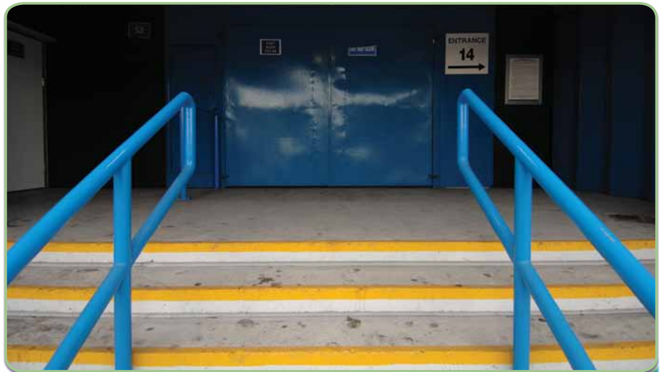
Figure 9 – Colour contrasting on steps
