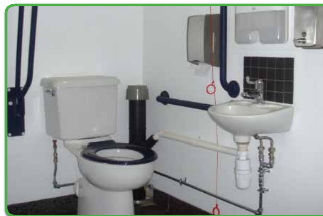
Figure 24 – An example of an accessible toilet
