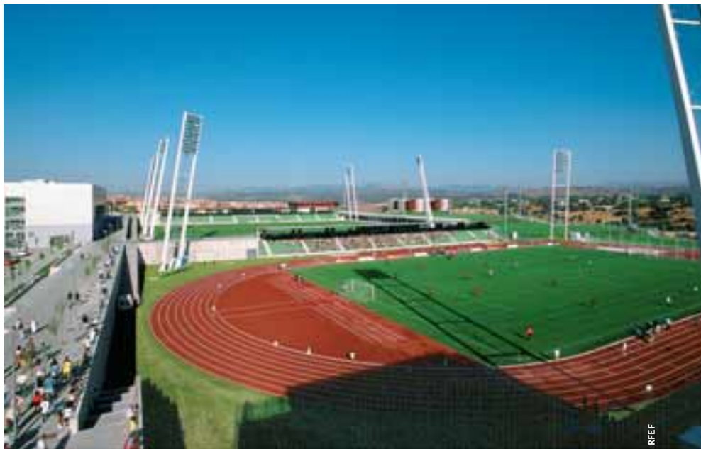
SPAIN The splendid facilities of Football City.
