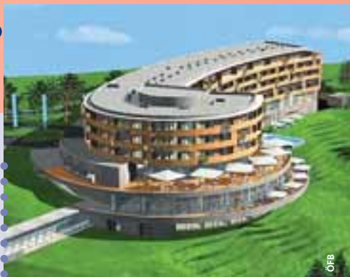
The facilities selected by Austria as the base for its national team during EURO 2008.
